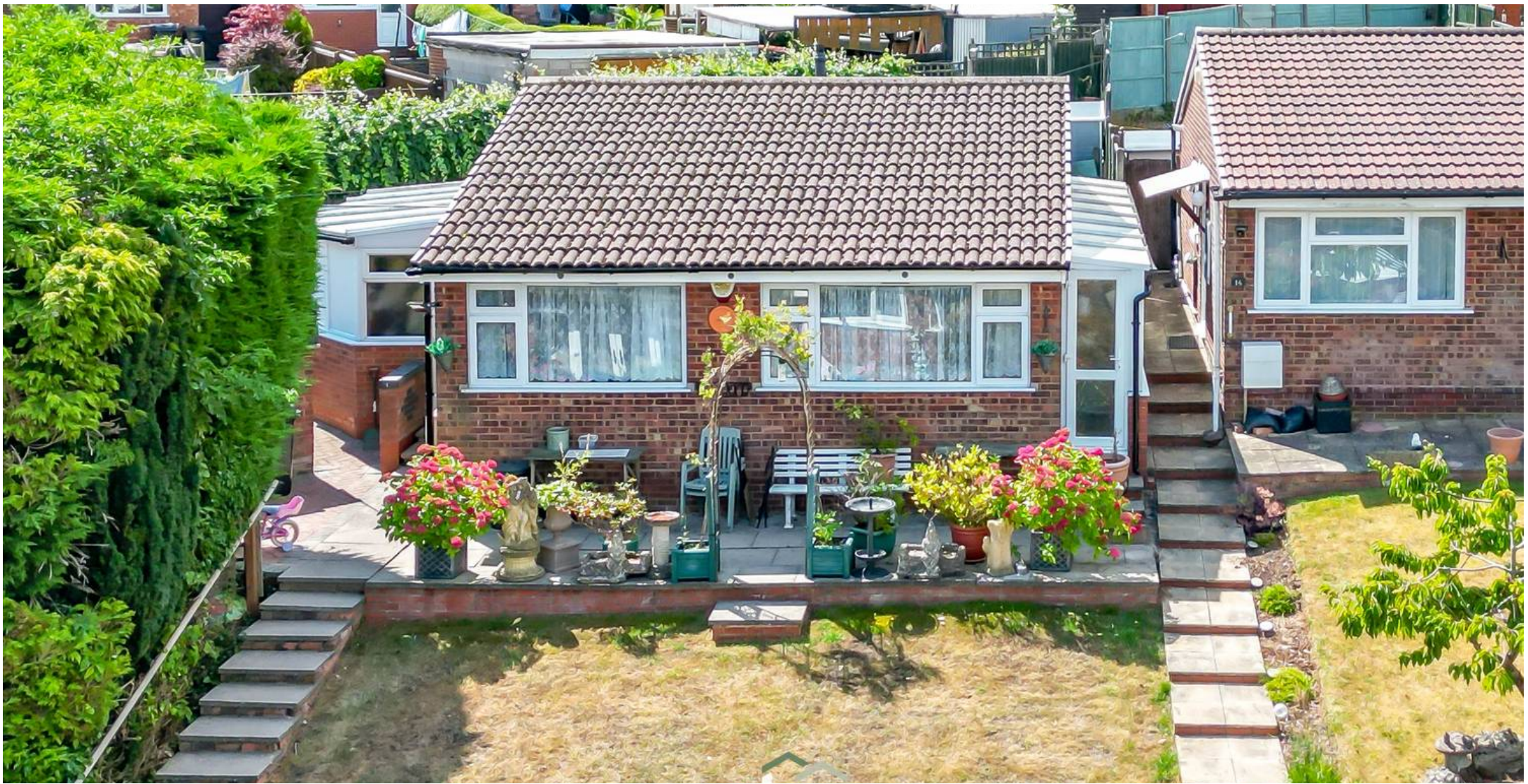
12 Heronfield Drive, Birmingham Birmingham
