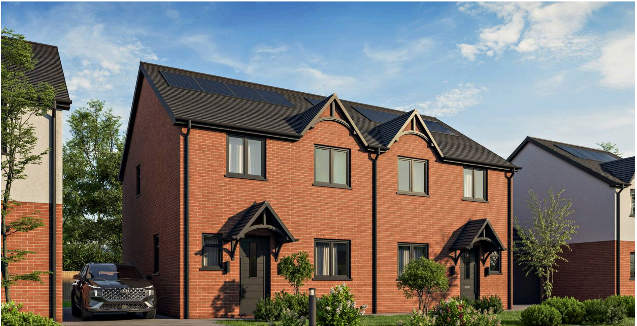
The Maple, Ailstone Mews, Old Birmingham Road Bromsgrove
